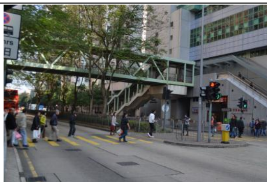
Picture B-5: Walkway bridge and cross walk at Yee Tai St.
