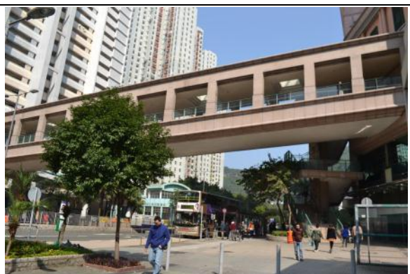
Picture D-3: Walkway bridge on Po Fung Rd.
