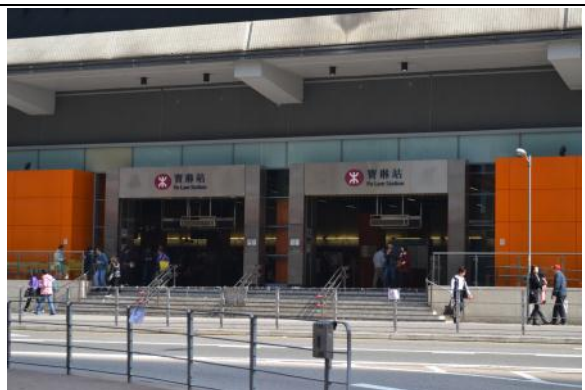
Picture D-1: Po Lam MTR Station
