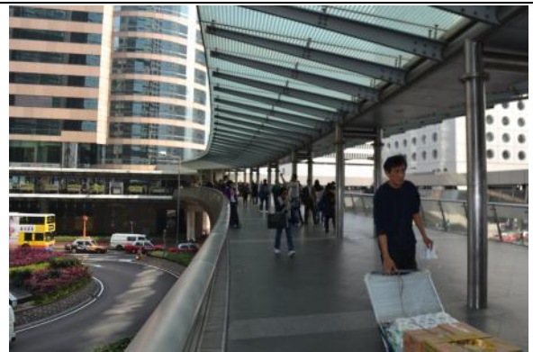
Picture A-4: Walkway bridge above Connaught Rd.
