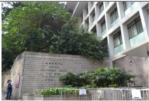
PictureA -14: Central Government Offices
