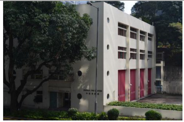
Picture A-16: Central Fire Station
