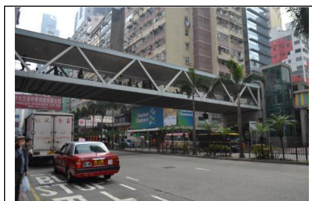
Picture E-2: Walkway Bridge on Hennessy Rd.
