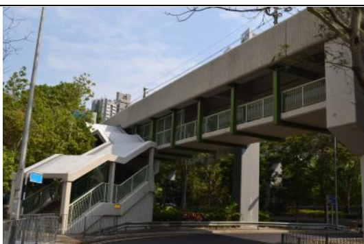
Picture B-2: Walkway bridge connected to MTR
