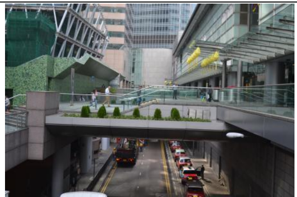
Picture A-5: Walkway bridge connecting to IFC Mall
