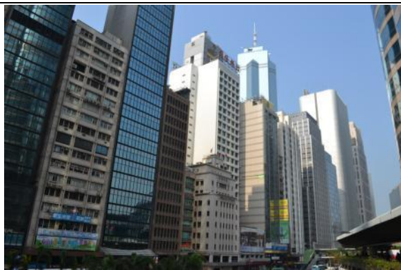
Picture A-9: Office buildings on Connaught Rd.
