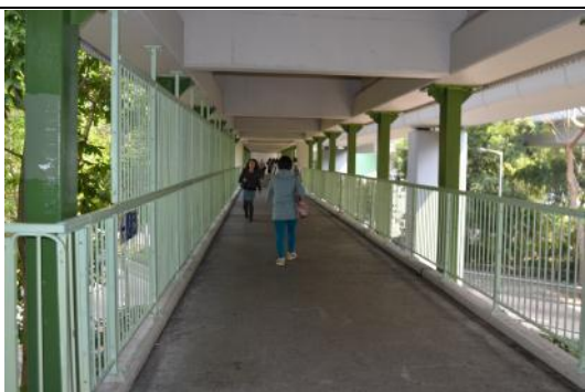
Picture B-3: Inside the walkway bridge
