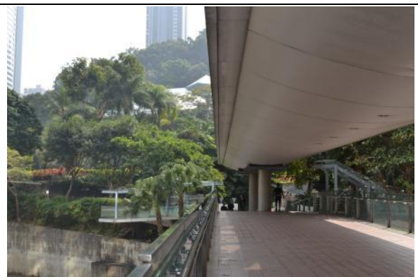
Picture A-6: Walkway bridge connecting to Hong Kong Park
