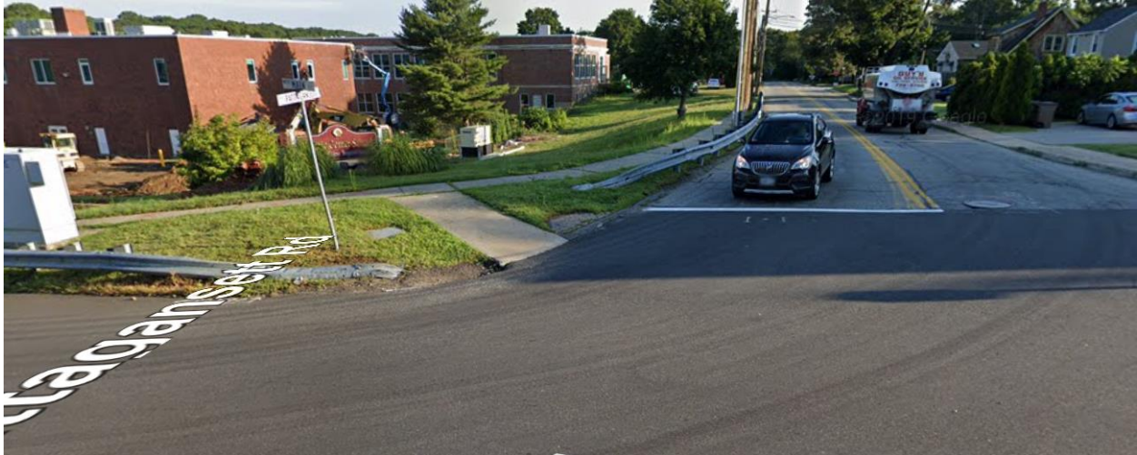
Figure 42: Google Earth view of Existing Condition of Curb Ramp i at Intersection A.
