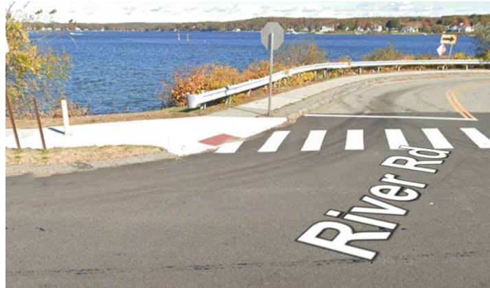
Figure 48: Proposed Google Earth view of Curb Ramp i at Intersection K in Zone 4.
