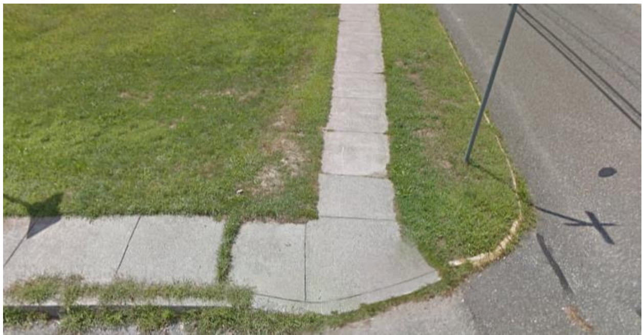
Figure 44: Google Earth view of Curb Ramp i at Intersection D in Zone 2
