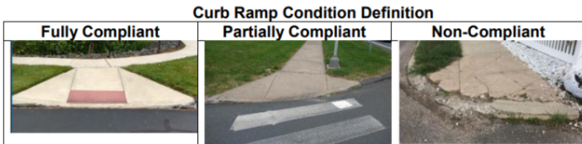
(Figure 3- Provides photos to demonstrate what sidewalks and curb ramps could look like with the corresponding categorization.)
