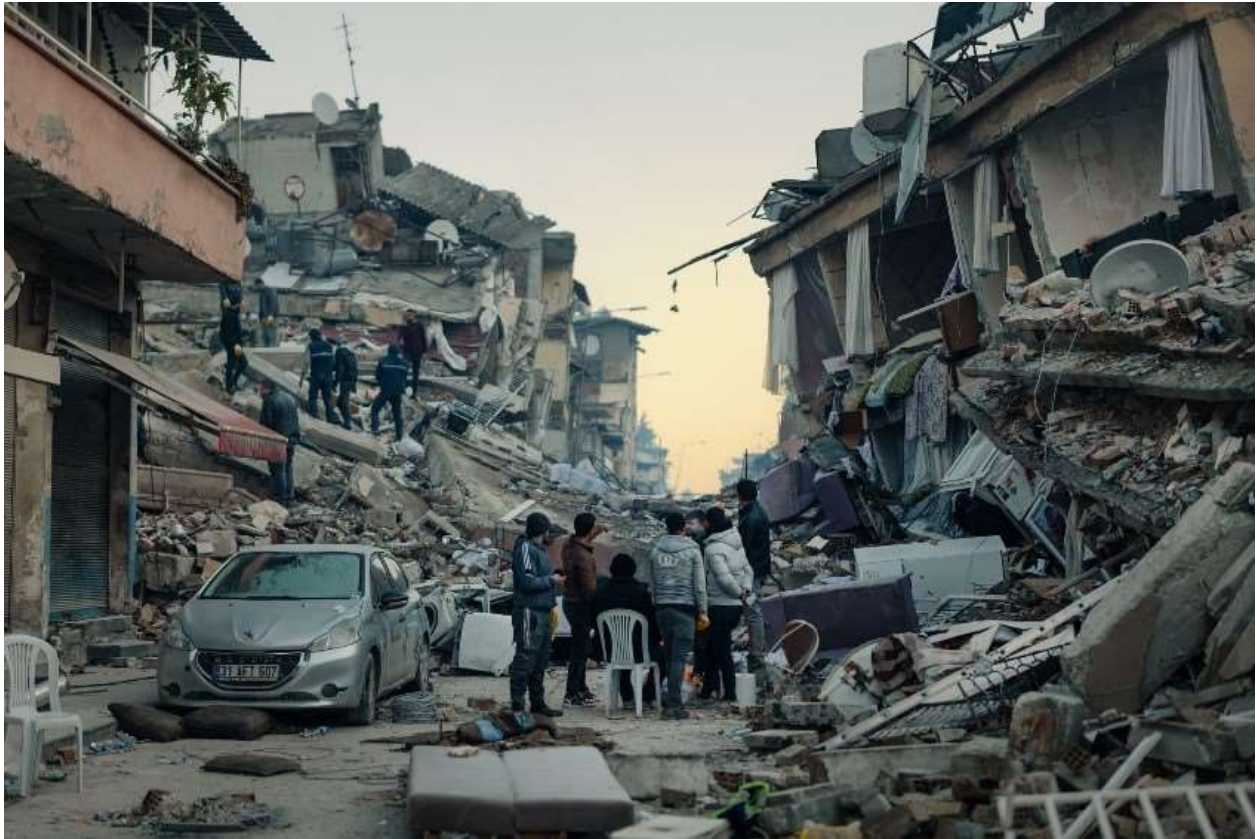
Figure 1: Damage in Ankara, Turkey (NY Times, 2023)
