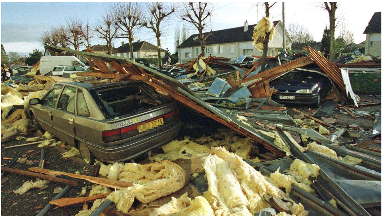
Figure 4: Damages from Storm Lothar, 1999 (Ouest France, 2019)
