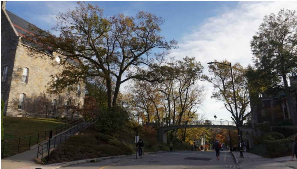
Figure 2: Existing Conditions, Earle Bridge. Photo courtesy of Worcester Polytechnic Institute (WPI, 2019).
