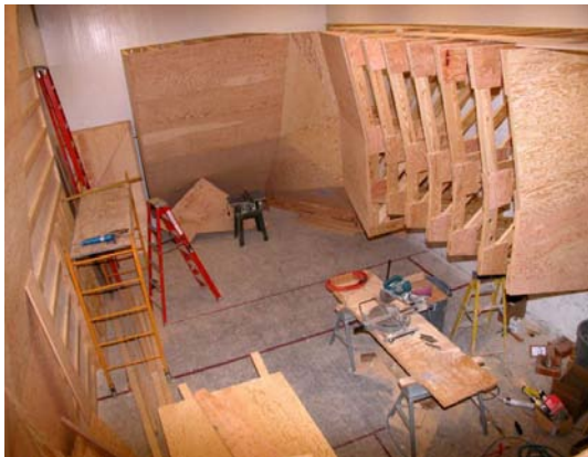
A bouldering wall under construction.
