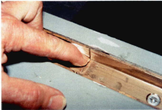
Picture 8: Rodney Hunt Manufactured Gate; tongue spacing
