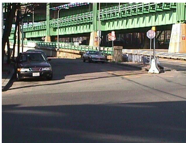
Figure 16 Beacon Street Off-Ramp Inclination
