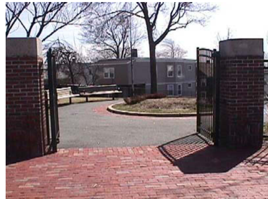
Figure 36 Entrance to Bellingham Hill Park
