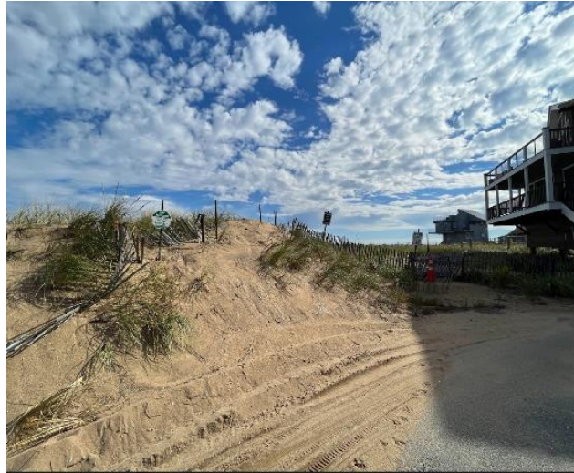
Figure 12. The former Newburyport pathway taken over by sand erosion.
