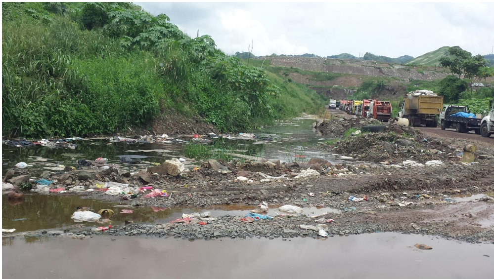
Figure 4: Leachate overflowing the road at Cerro Patacón
