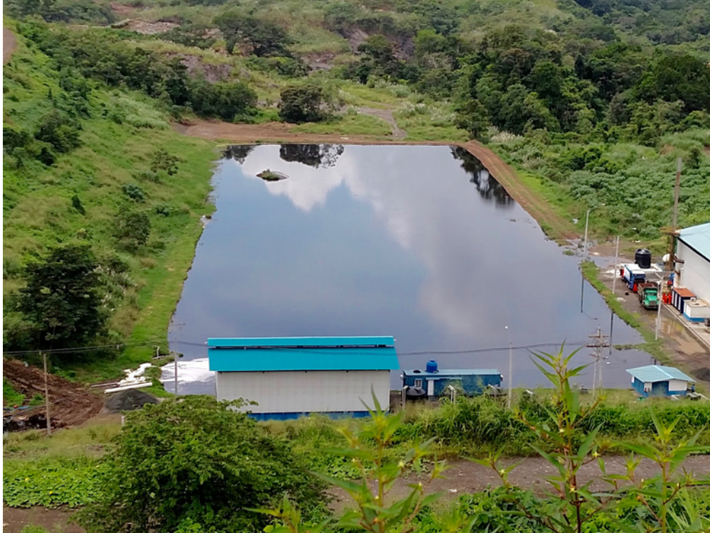
Figure 3: Flooded leachate treatment pools at Cerro Patacón
