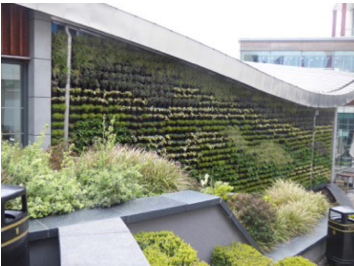
Figure 8: Living Wall. A living wall installed on the outside wall of a building. (Flickr, 2018)
