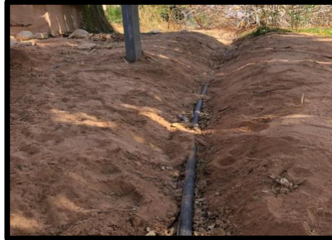
Figure 4.4 The new trench
