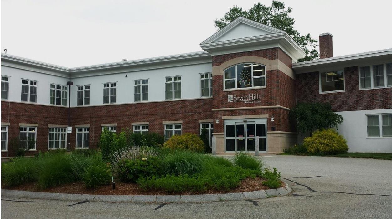
Figure 1: Seven Hills Pediatric Center, located in Groton, Massachusetts.
