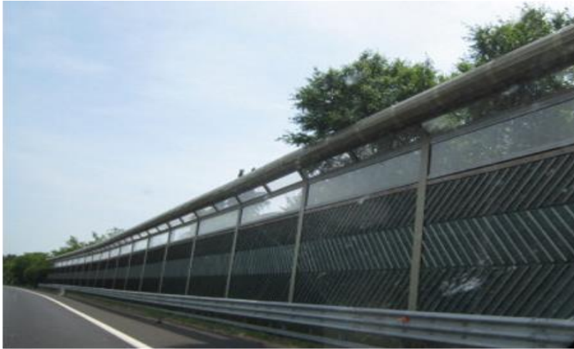
Figure 1: A noise reduction capped barrier on the side of a highway (Murphy & King, 2014)
