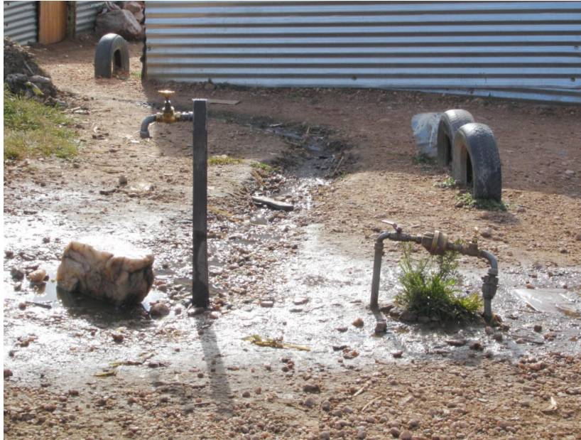
Figure 6: Post-pay Standpipe and Meter
