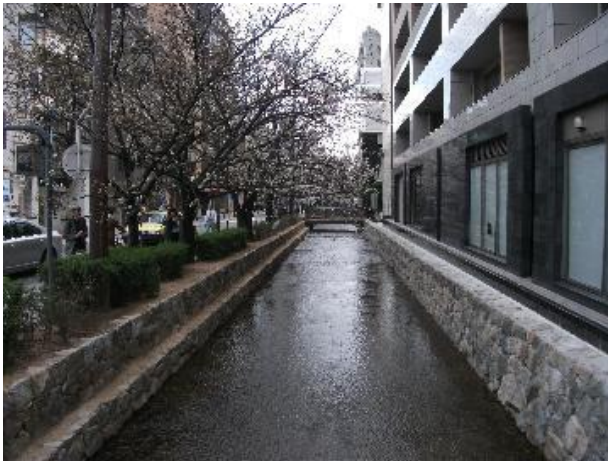
Figure 6: Oike-dori after repairs
