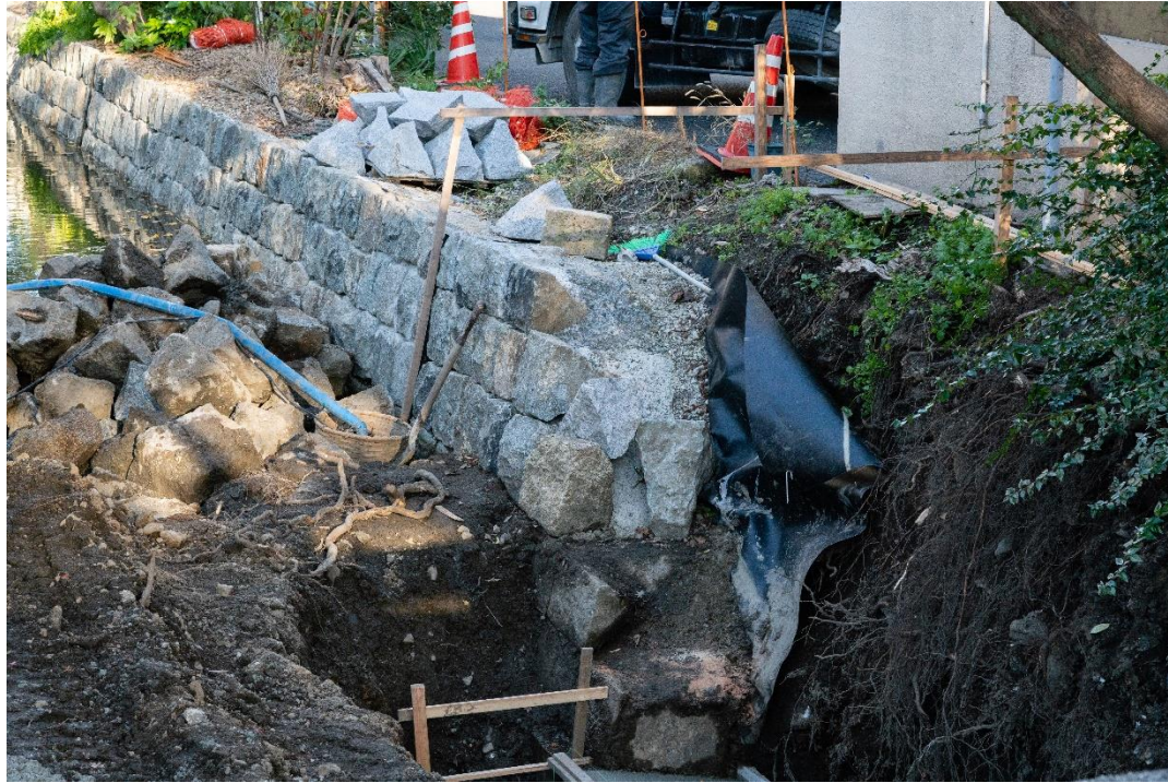
Figure 4: Waterproof sheets being placed behind rocks
