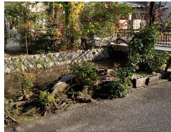
Figure 50: Image of tree that was removed after falling
