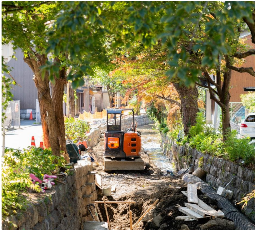
Figure 1: Current Restoration in Kikuhama Region
