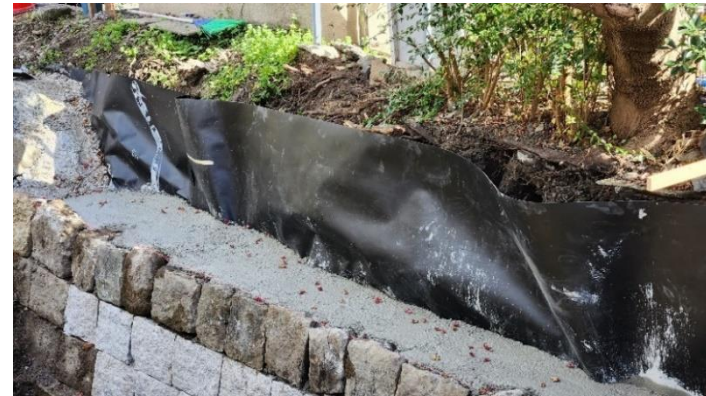
Figure 22: Face Rock Repair Without the Removal of Vegetation
