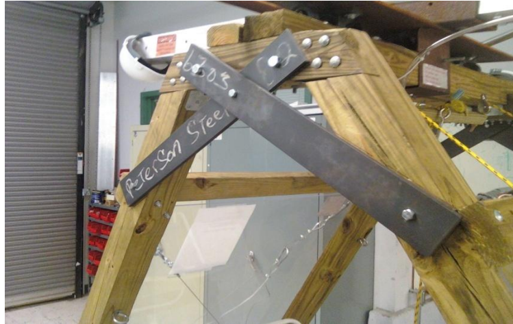
Figure 34 - A-frame with added cross reinforcement
