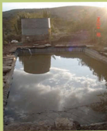
reservoir at Kimbo School.
