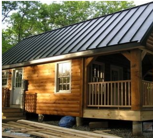
Figure 16: Example of Corrugated Roof on a Cabin (Riverside Sheet Metal, 2019)
