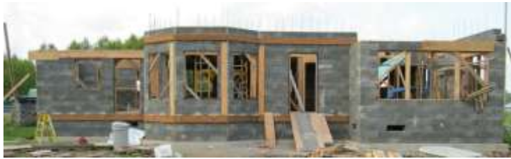
Figure 30: FasWall Project in Progress (FasWall Home)
