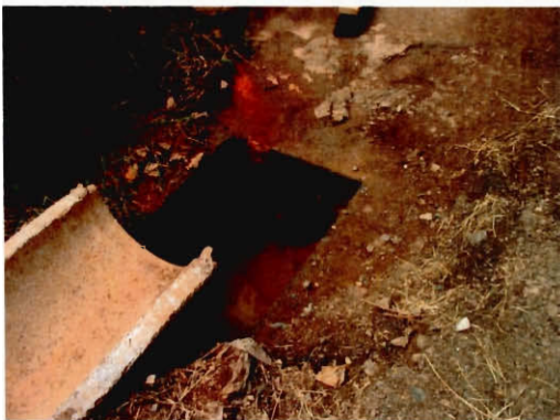
Figure 3: Stream Collection Reservoir
