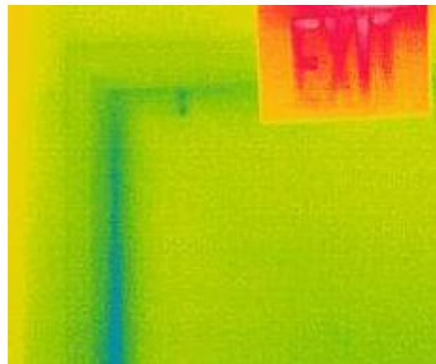
Figure 8: Properly Sealed Door
