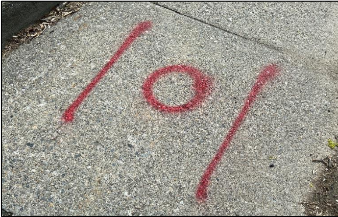
Figure 20: Example electrical marking
