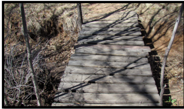
Figure 22: Bridge on Calle Lorca Trail
