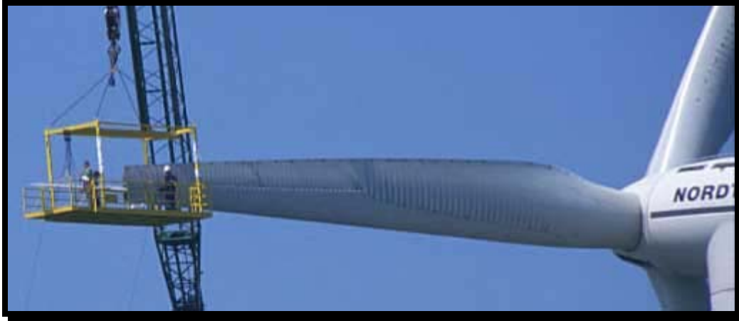
Figure 5.3: Repairs being made to an industrial-size blade
