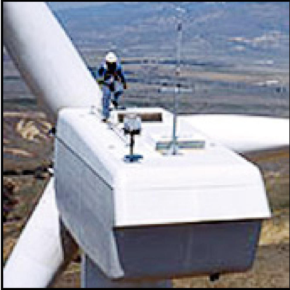
Figure 2.2: Utility Scale Wind Turbine
