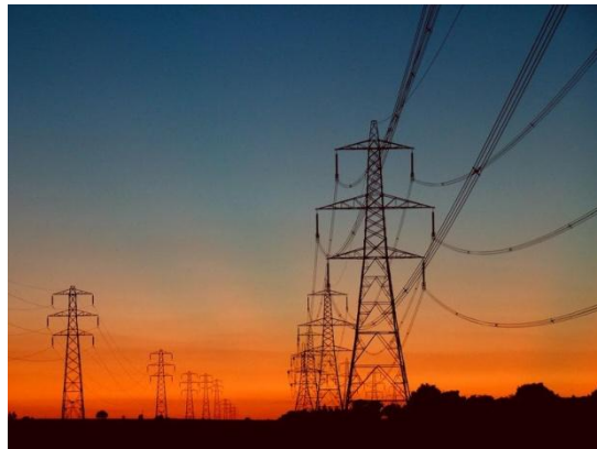
Figure 2: Overhead Electrical Power Lines
