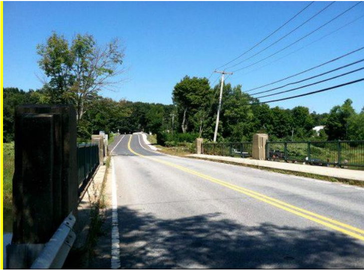
Figure 1 - Dip between Existing Bridge and CSX Bridge
