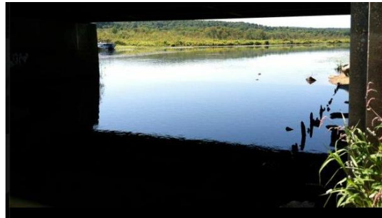
Figure 4: Downstream from the Bridge
