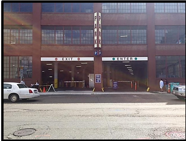
Causeway Street entrance to the North End Garage (Ian Smith, 2016).
