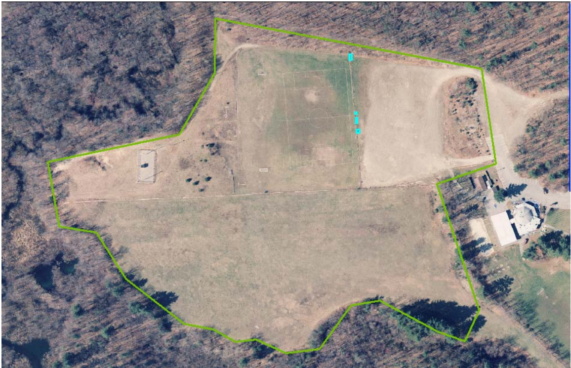
Figure 63: Lake Street Recreation Area Structures
