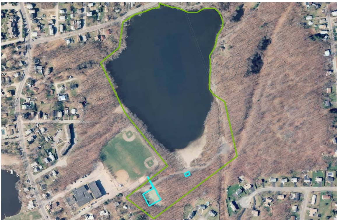
Figure 58: Jordan Pond Structures
