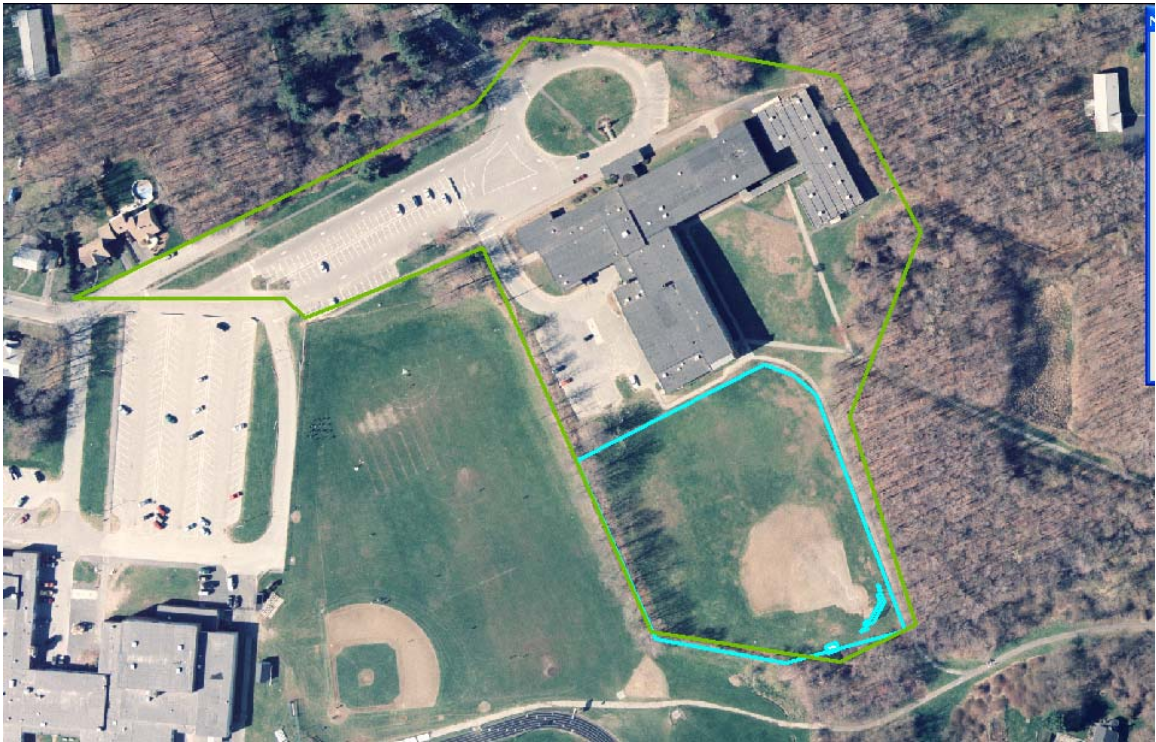
Figure 89: Sherwood Middle School Structures
