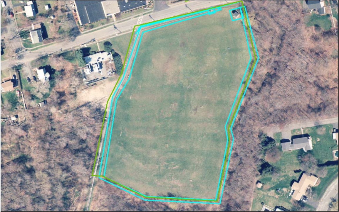
Figure 72: Municipal Drive Structures
