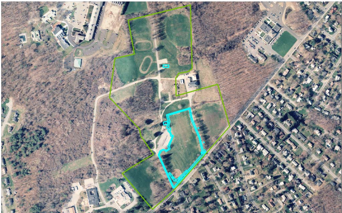
Figure 67: Maple Avenue Structures
