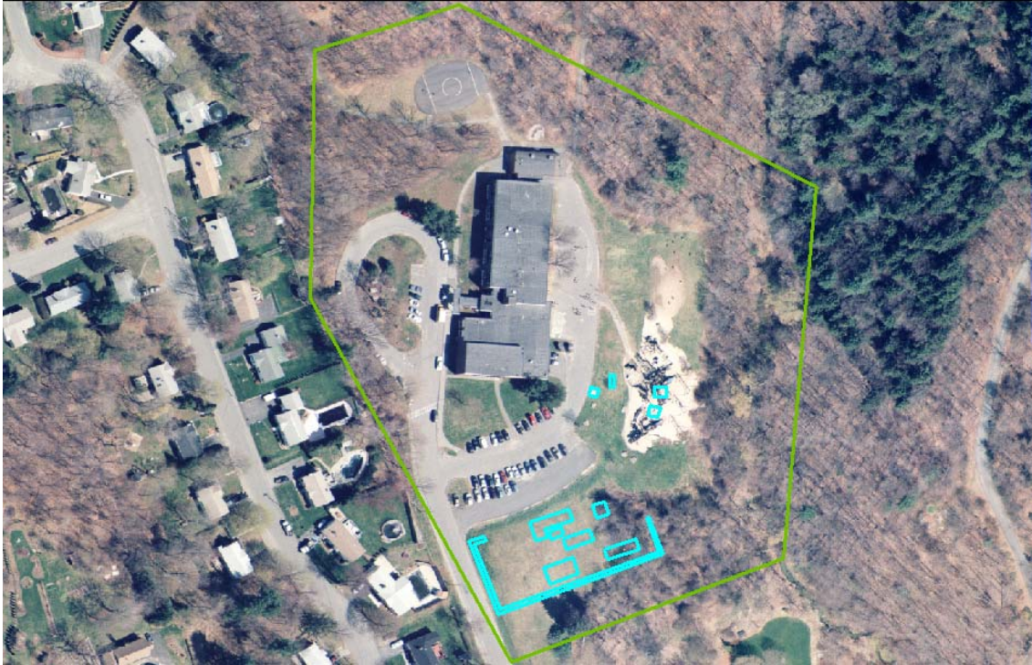
Figure 92: Spring Street School Structures
