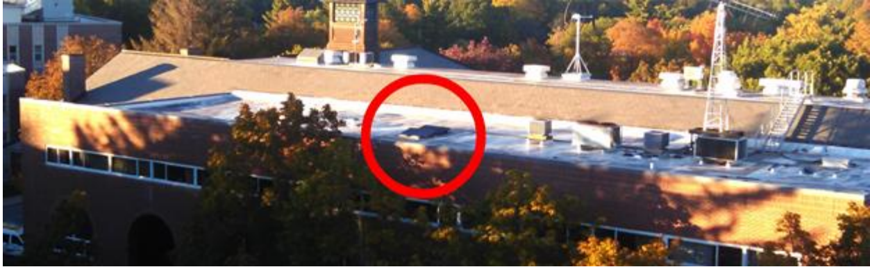
Figure 2. Location of Solar Panels on roof of Atwater Kent
