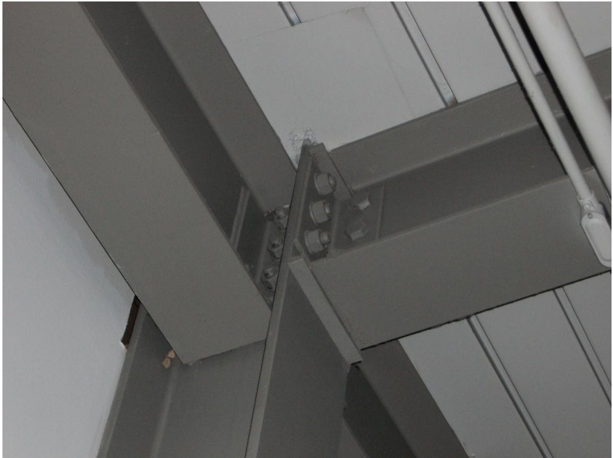
Figure 31: Photo of a Sample Bolted Connection in Fuller Labs at WPI
