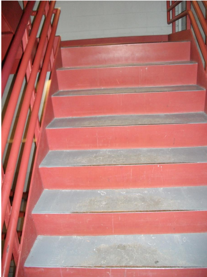
Figure 33: Stairs with Concrete-Filled Steel Pans
