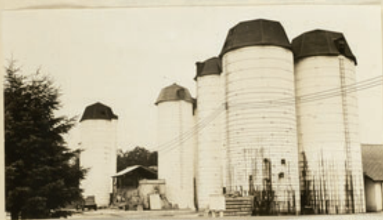
SILOS AT SUSSEX NEW JERSEY
