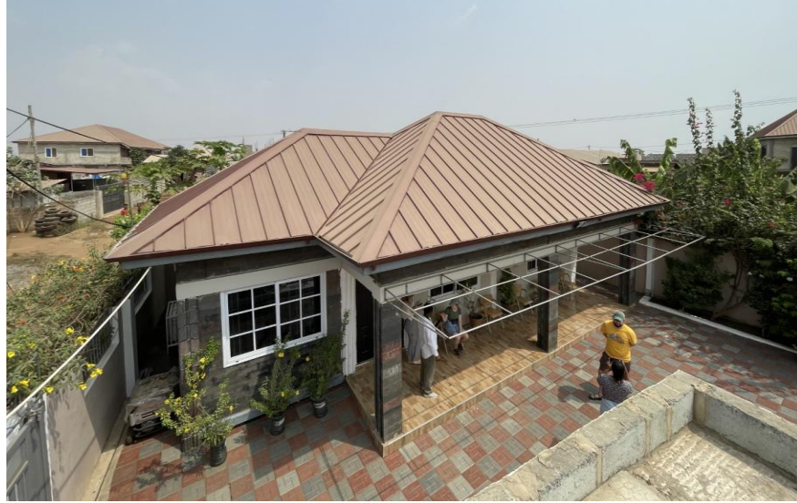
Figure 5: Nelplast Eco's prototype home built entirely from Eco Blocks (excluding the roof). Photo Credit: Michael Morin
