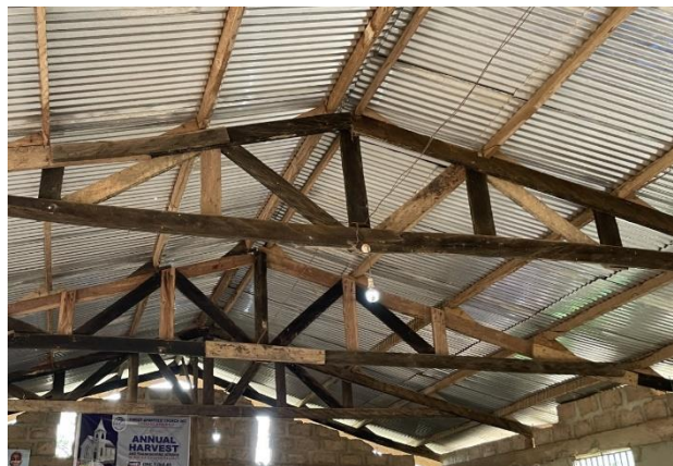
Figure 28: Photo of wooden roofing trusses at a church in Akyem Dwenase. Photo Credit: Michael Morin
