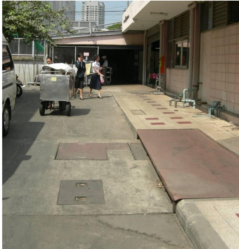
Figure 17: Uneven Surfaces Which Trolley Has to Travel Over
