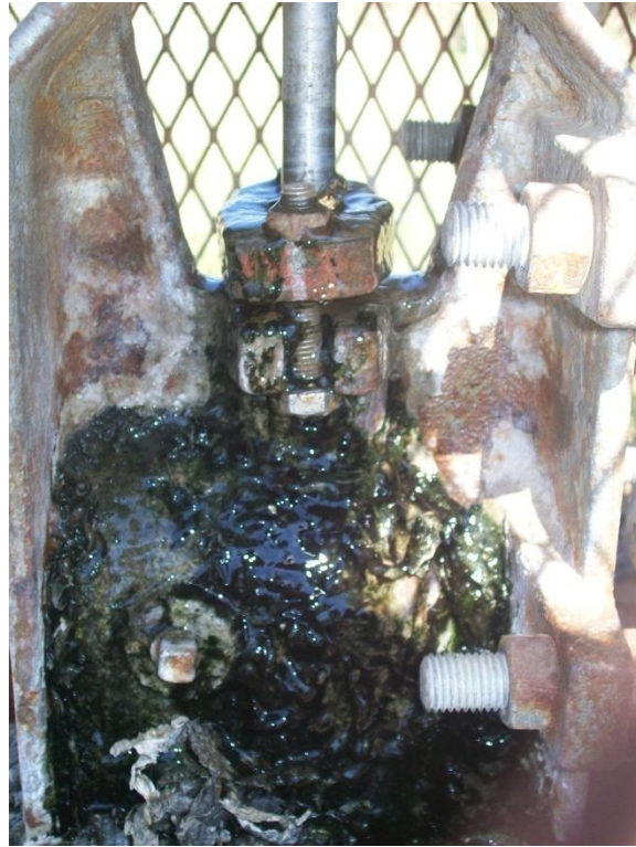
Figure 35- Leaking water pump in Drimiopsis
