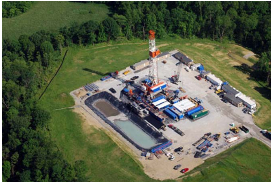
Figure 3.4: Drilling site in the Marcellus xxxiv
