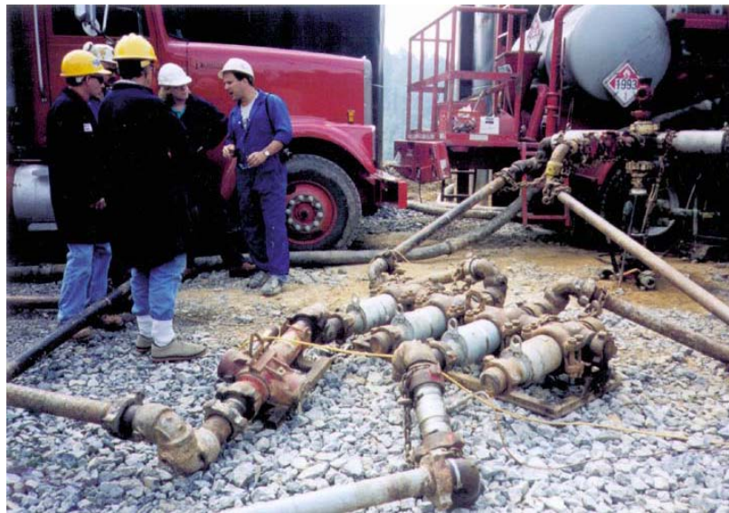
Figure 3.2: The fracturing fluids, additives, and proppant are pumped to the wellhead and mixed just prior to injection. xxxvii
