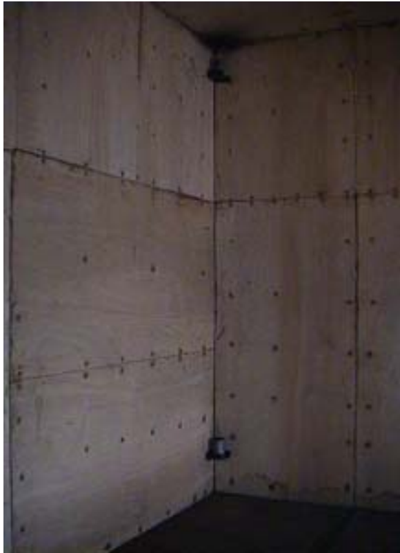
Photograph 5. Inside of Enclosure
