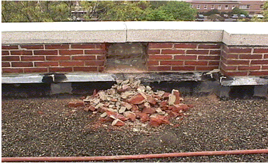
Figure 2.3. Removal of masonry blocks and roof caps for roof membrane replacement
