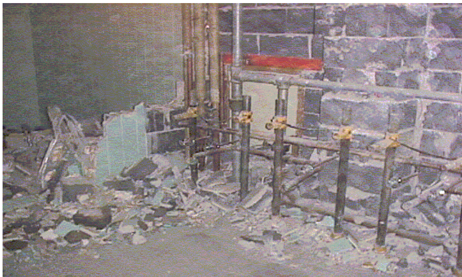
Figure 2.4. Plumbing pipes ready to be replaced
