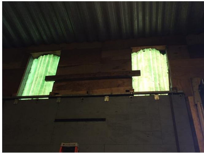
Figure 9: Converted Gymnasium in HQ Garage
