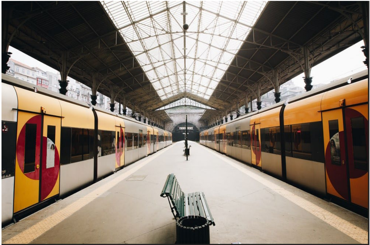
Figure 51. Train background. Source: URL
