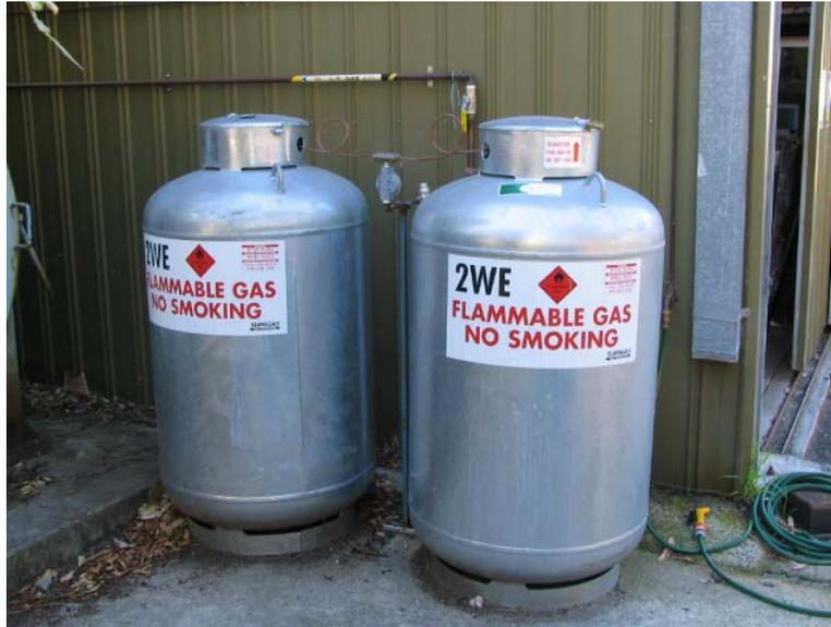
**Figure 3-1 LPG Gas Containers Used with Radiant Panel Array**
