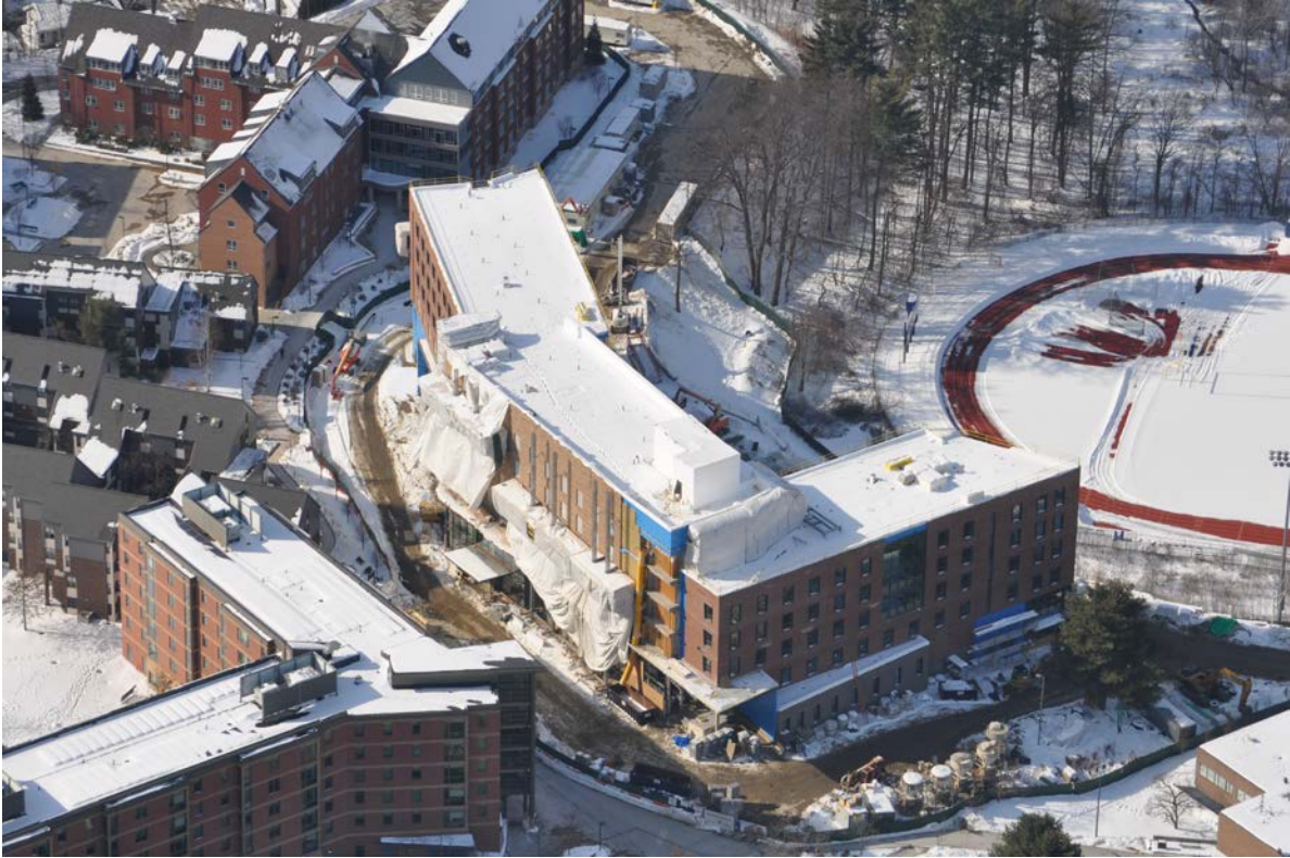
Figure 52: Site Overview - February 2014
