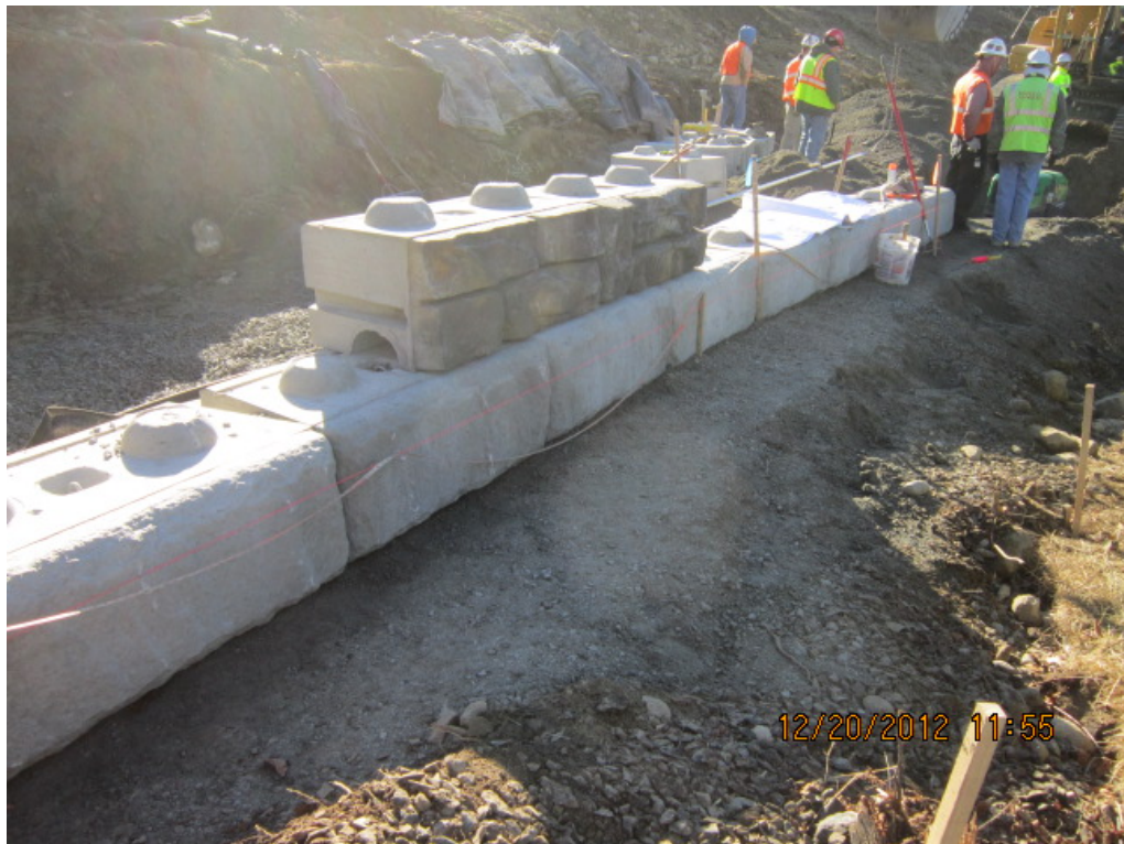
Figure 39: Retaining Wall Construction - December 2012
