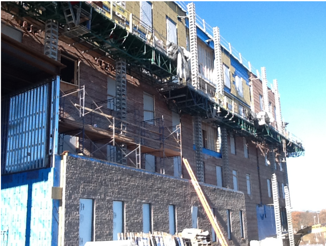
Figure 49: Masonry (Wing 1) - November 2013
