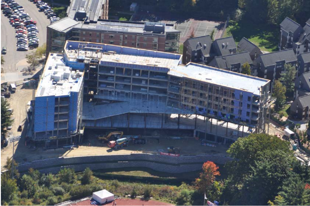
Figure 48: Site Overview - October 2013
