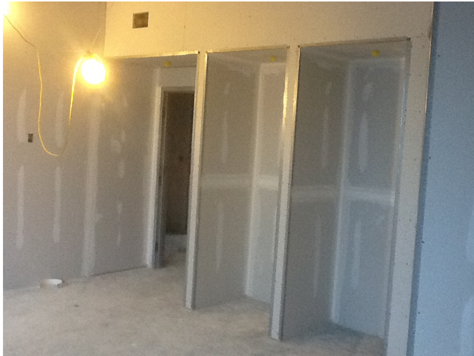
Figure 51: Interior Finishes - January 2014
