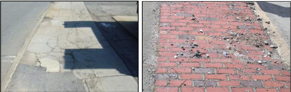
**Figure 12: Cracked Sidewalk (left); Poorly maintained brick (right)**
