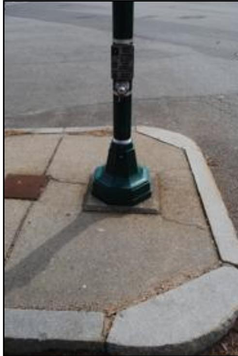
**Figure 27: Walking light located on top of an inaccessible median at the intersection of Langley Road and Beacon Street**
