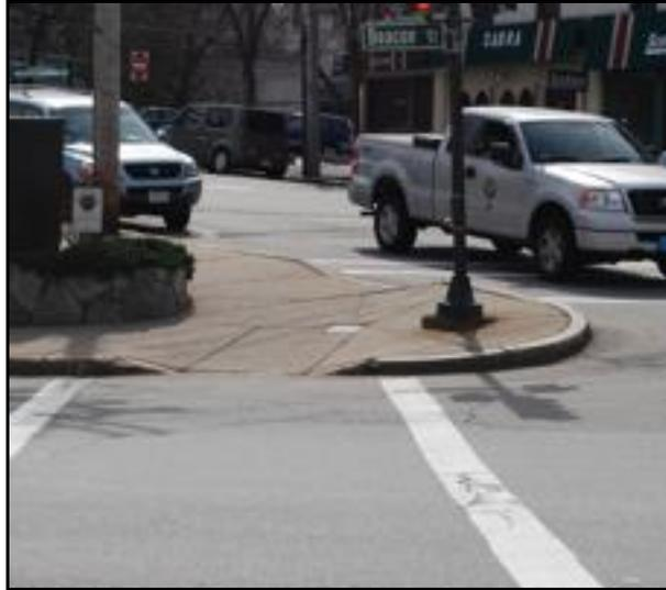
**Figure 28: Steep curb cut located at the intersection of Langley Road and Beacon Street**
