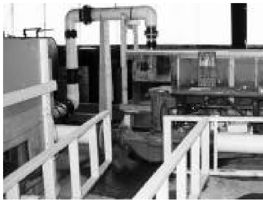
Figure 3-3: View of Tank Intake
