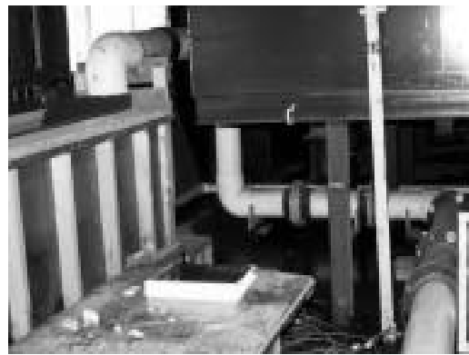
Figure 3-4: View of Tank Inlet
