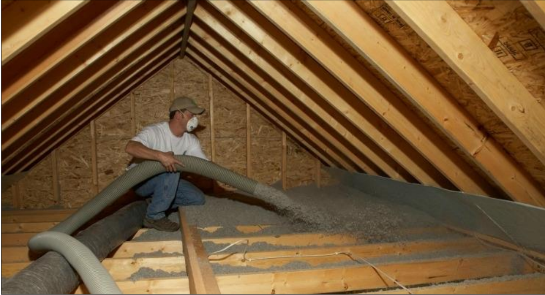
Figure 2.1-2: Blown-in insulation of cellulose (USDOE, Energy Saver, 2013)
