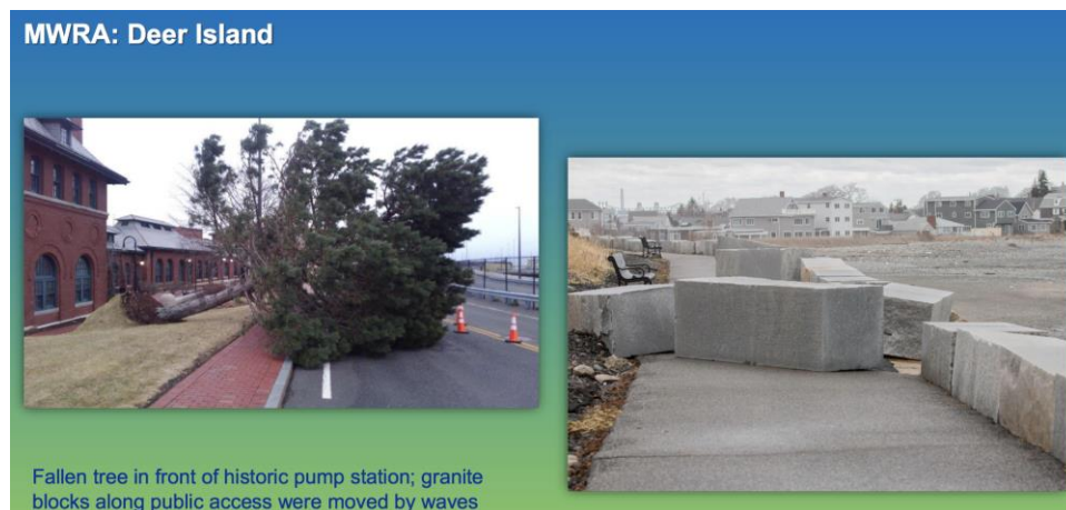
Figure 5: Storm Damage to Deer Island
