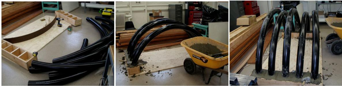
Figure 5 - Footing Form (L), Poured Footing (C, R)
