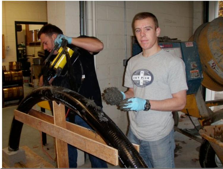
Figure 6 - Inserting Concrete in to Top of Arch and Use of Mechanical Vibrator
