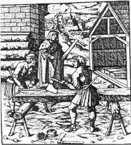
Figure 10 Squaring a piece of timber with an axe. (From Singer, 1956)
