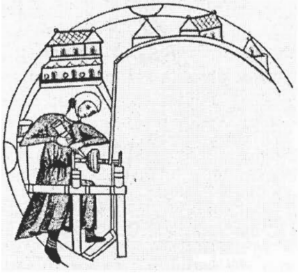
Figure 19 Turning a wooden bowl on a pole lathe. (From Singer, 1956)
