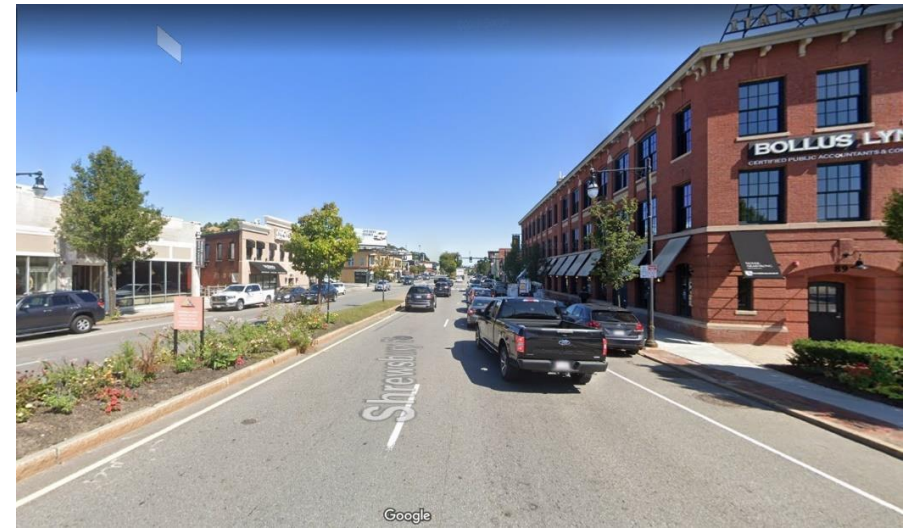
Figure 16: Shrewsbury Street commercial area (Google Maps, 2020)
