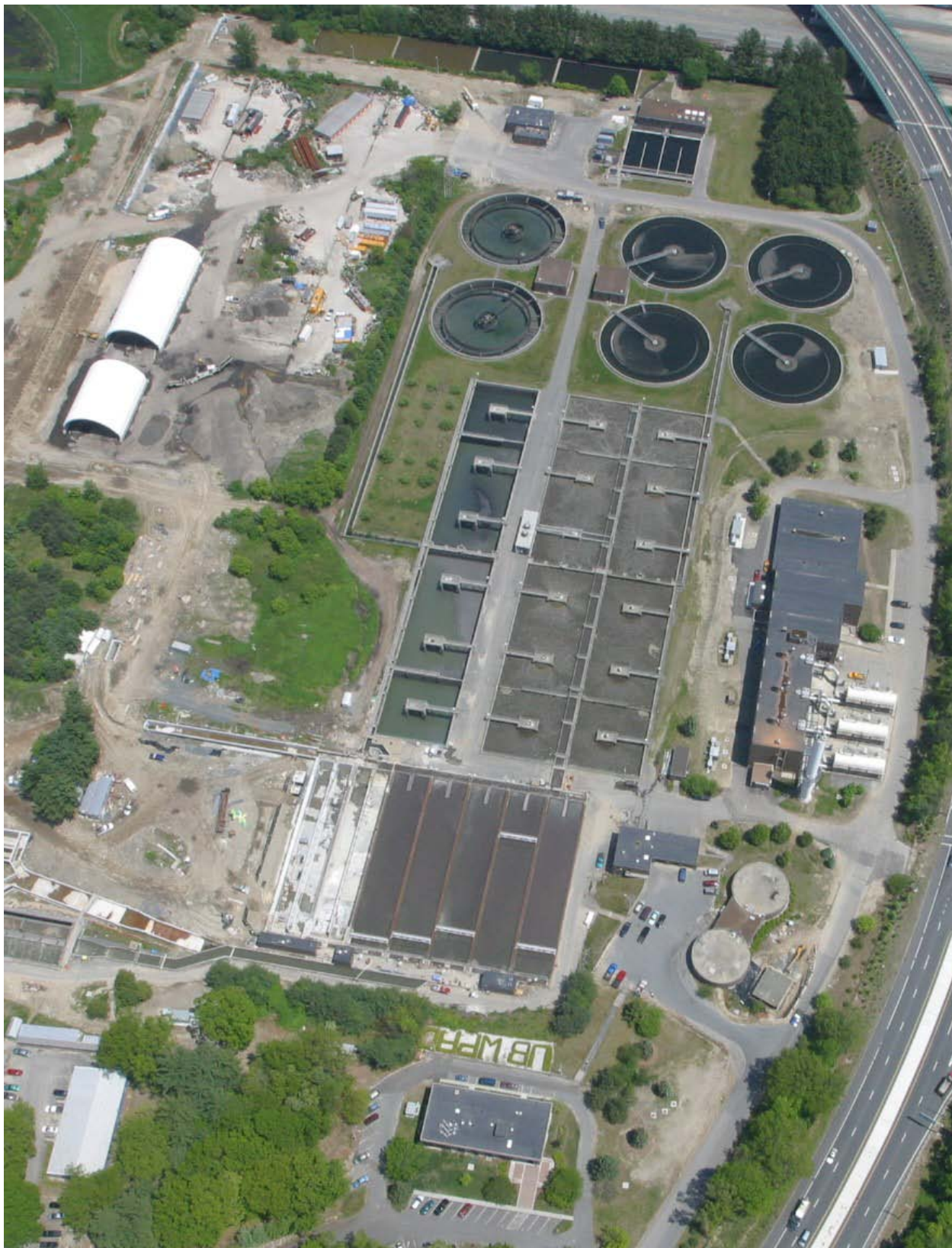
Figure 4-1: Aerial view of the Upper Blackstone Water Pollution Abatement District in Millbury, MA (Source: www.wbpad.org )
