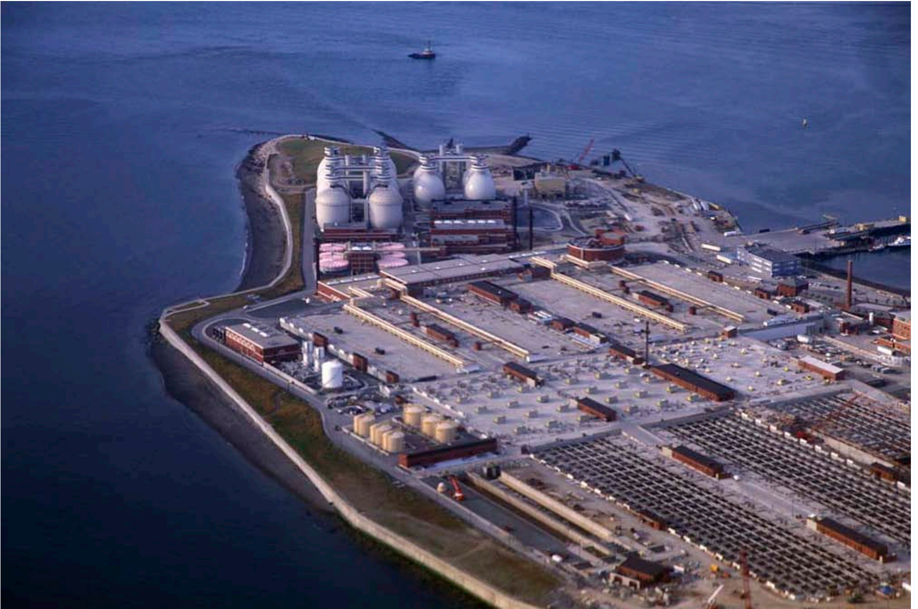
Figure 3-1: Deer Island Water Treatment Plant, Boston, MA (Source: Dan L. Perlman, www.ecolibrary.org )
