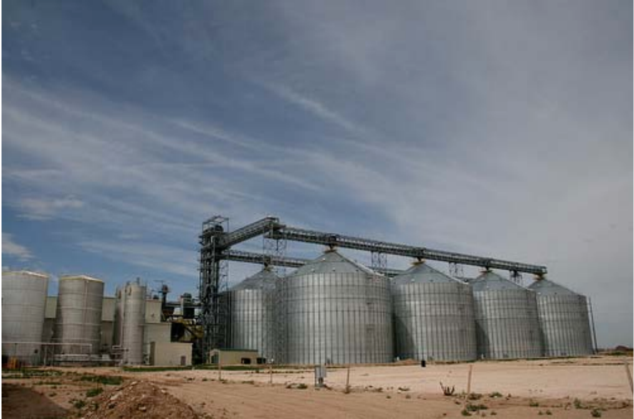
Figure 4-2: Panda Energy International Facility in Hereford, TX (Source: http://www.bbc.co.uk/worldservice/news/2009/06/090623_ethanol_wt_sl.shtml , 04/10/10)
