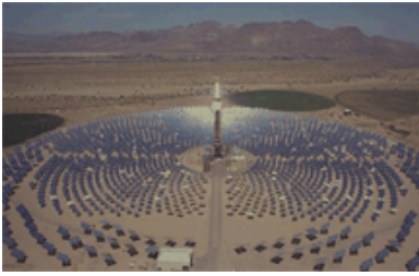
Figure 29: Power Tower and Field of Heliostats *
